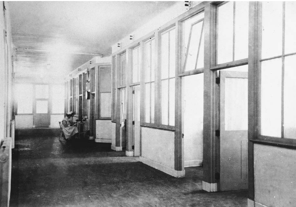
FIGURE 2.20. Glass screens at Hôpital Ste-Justine, Montreal, combined the need for segregation and surveillance.
