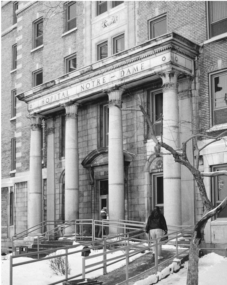
FIGURE 5.1. Stevens and Lee's entrance to Hôpital Notre-Dame featured classical columns.
