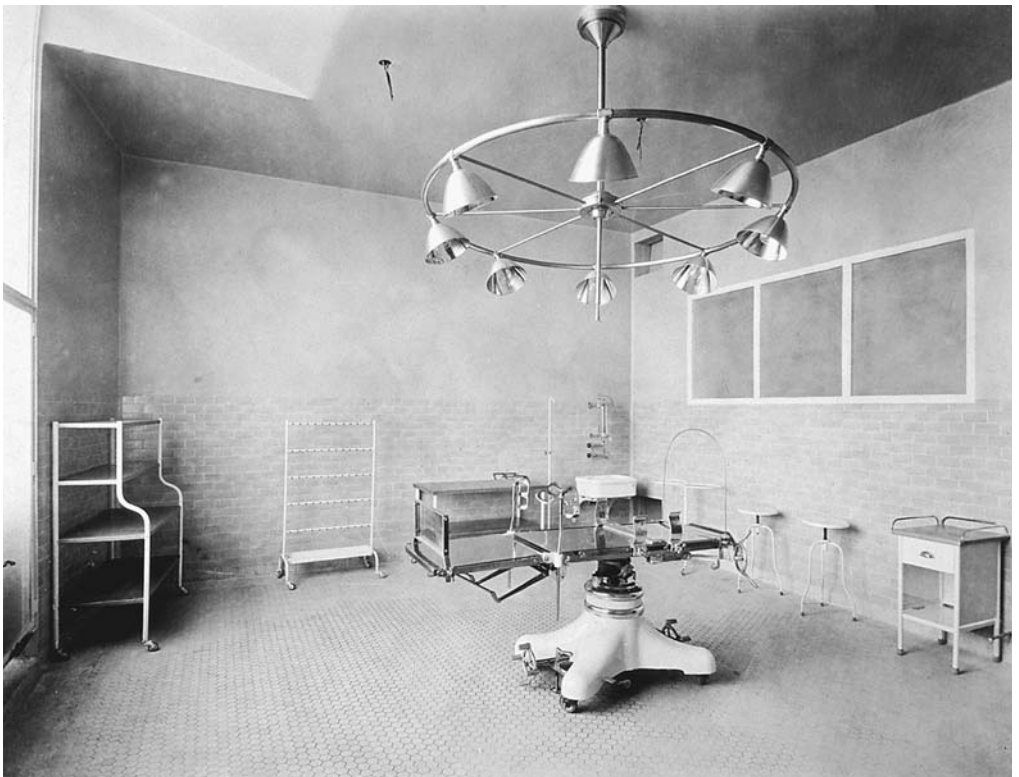
FIGURE 5.16. Delivery room, Ottawa Civic Hospital, 1926.
