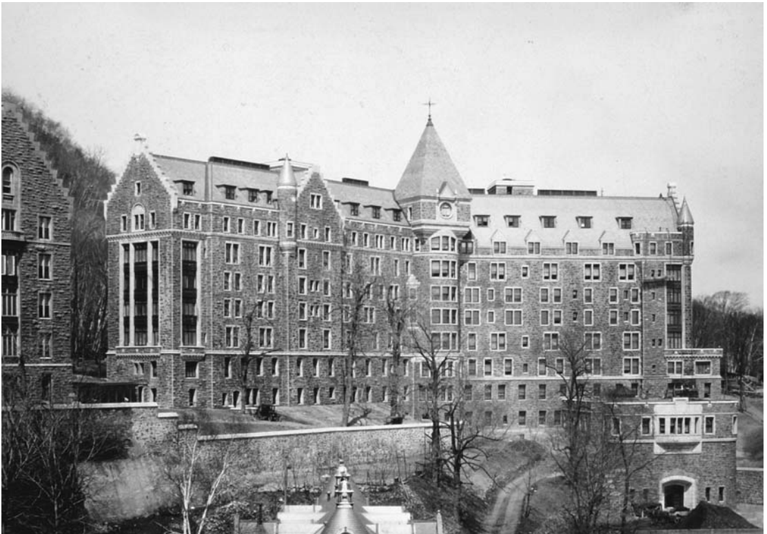
FIGURE 2.13. Royal Victoria Montreal Maternity Hospital.
