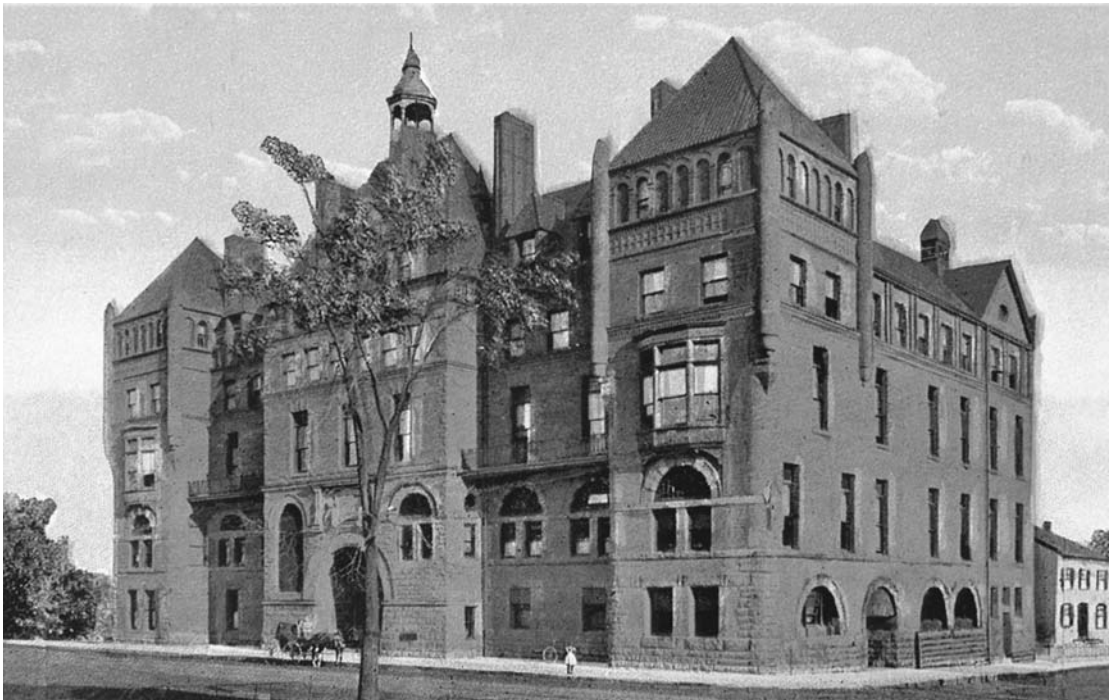
FIGURE 2.18. The Victoria Hospital for Sick Children, Toronto, resembled a grand railway hotel.
